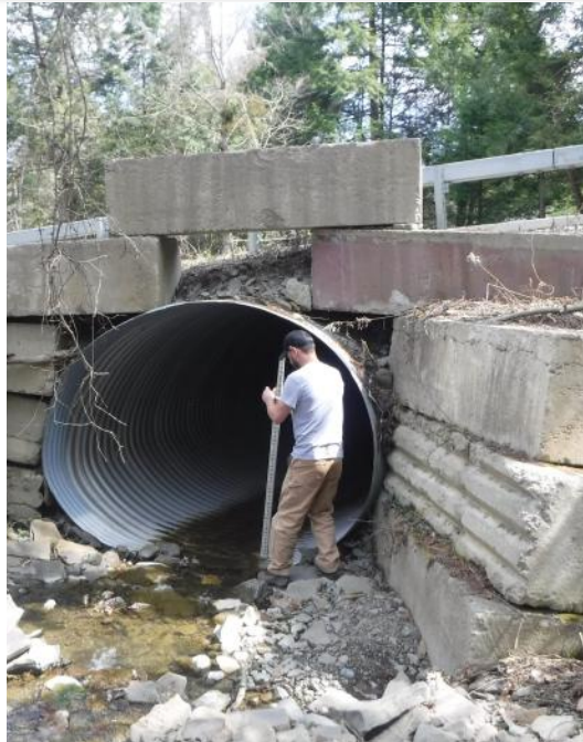
Performing culvert assessments for municipalities in 2021.
