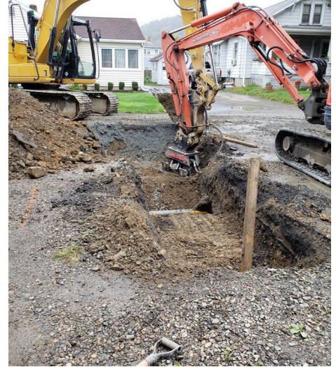
Leland Street Area Sanitary Sewer Town of Southport, NY
