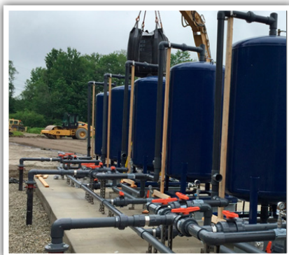
Photo left: Six granulated activated carbon treatment units. Photo right: Gary Ginsberg, Adam Helman and Daniel Lang, NYSDOH; Shawn Ecklund and Samuel Ambrose Village of Mayville, and Casey Miller, Chautauqua County Department of Health and Human Services.
