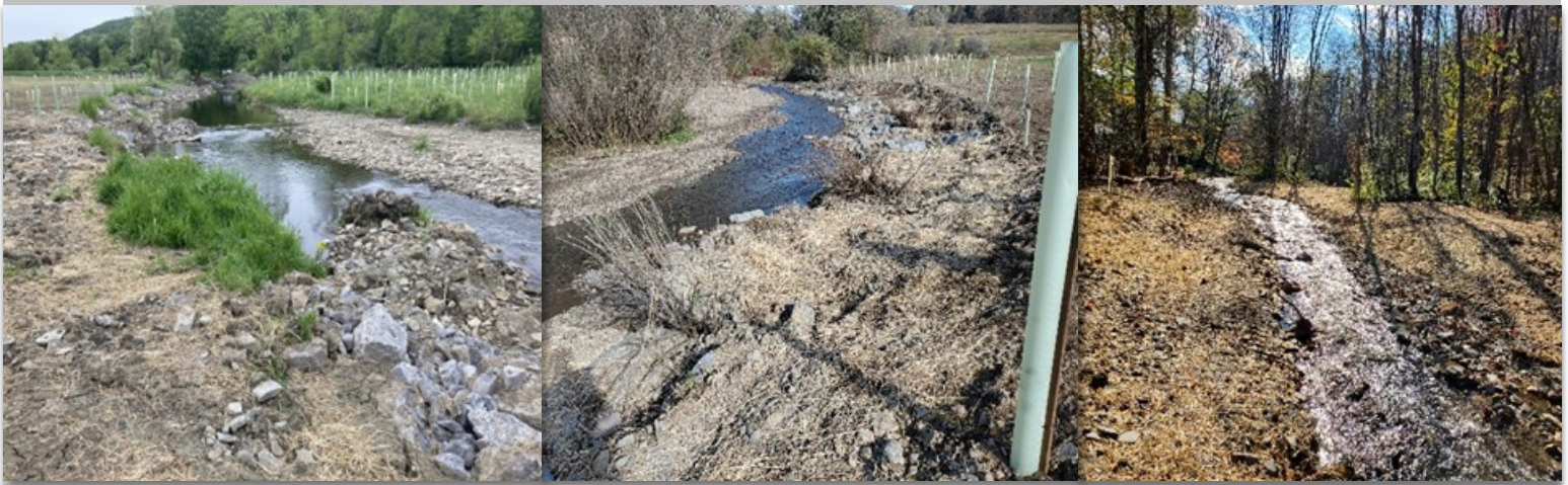
Streambank Protection Projects in Cortland County (above)
